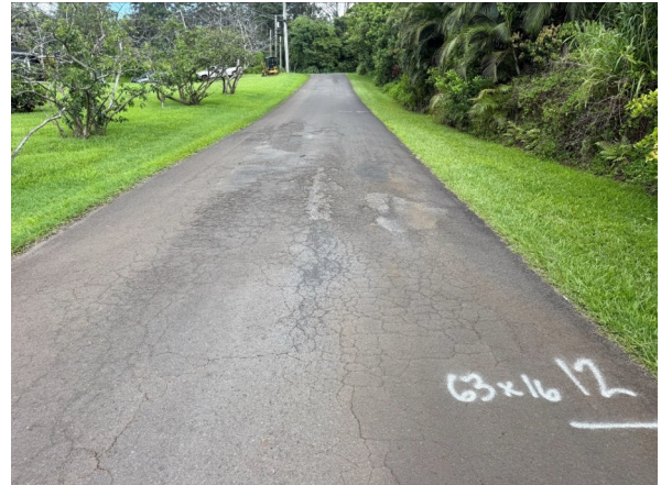
One of the fifteen surveyed areas, measured and marked on the pavement.
