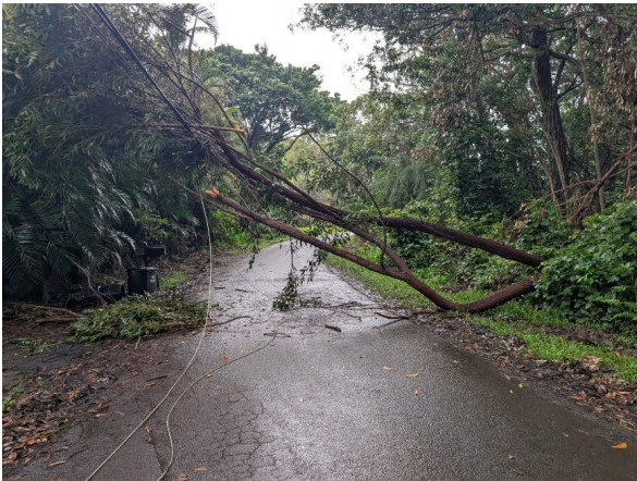
Storm cleanup: a tree down across the road, with a utility line pulled down alongside it.
